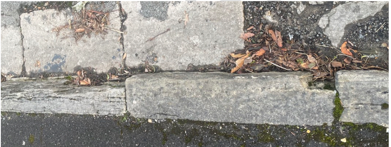
Purbeck kerb and white limestone gutter stones in Leigh Road
