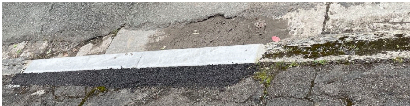
Leigh Road concrete replacement
