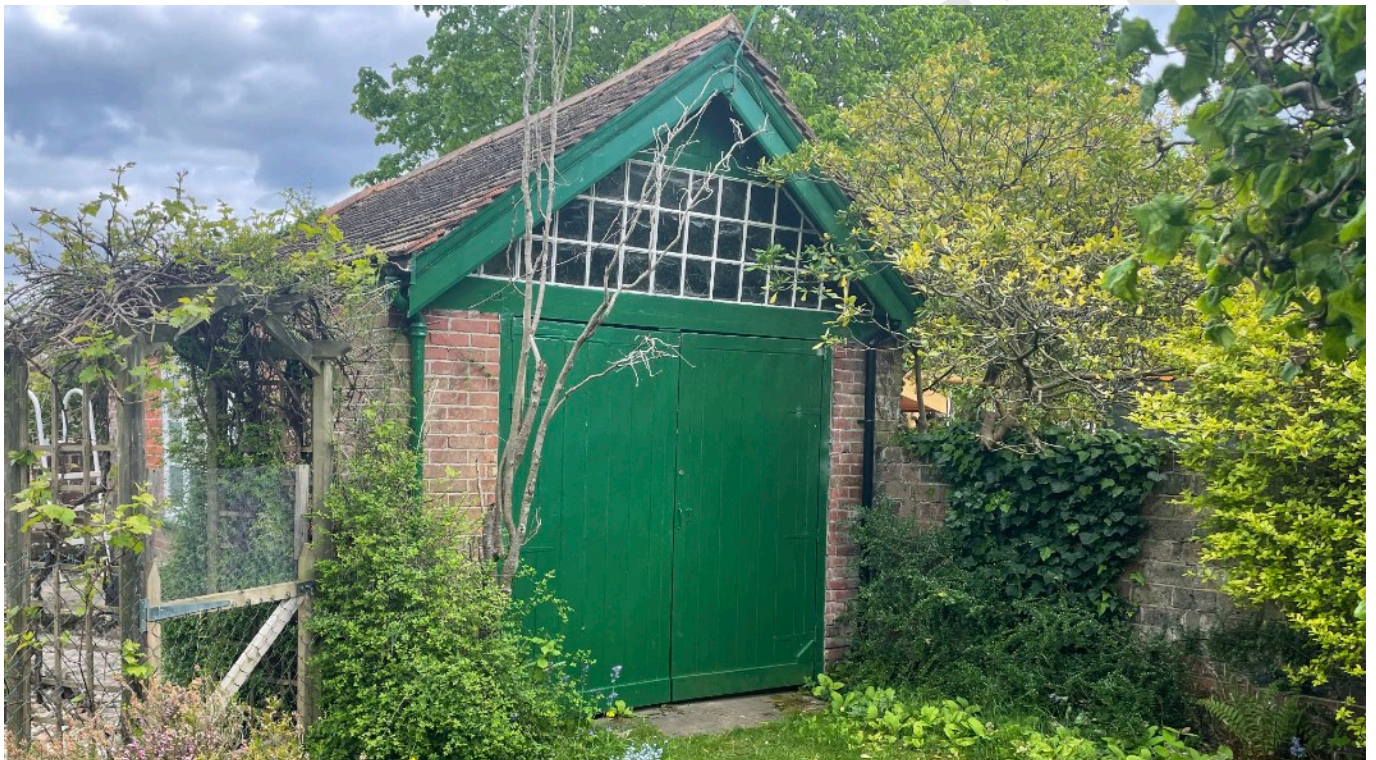
1913 “motor house” in back garden
